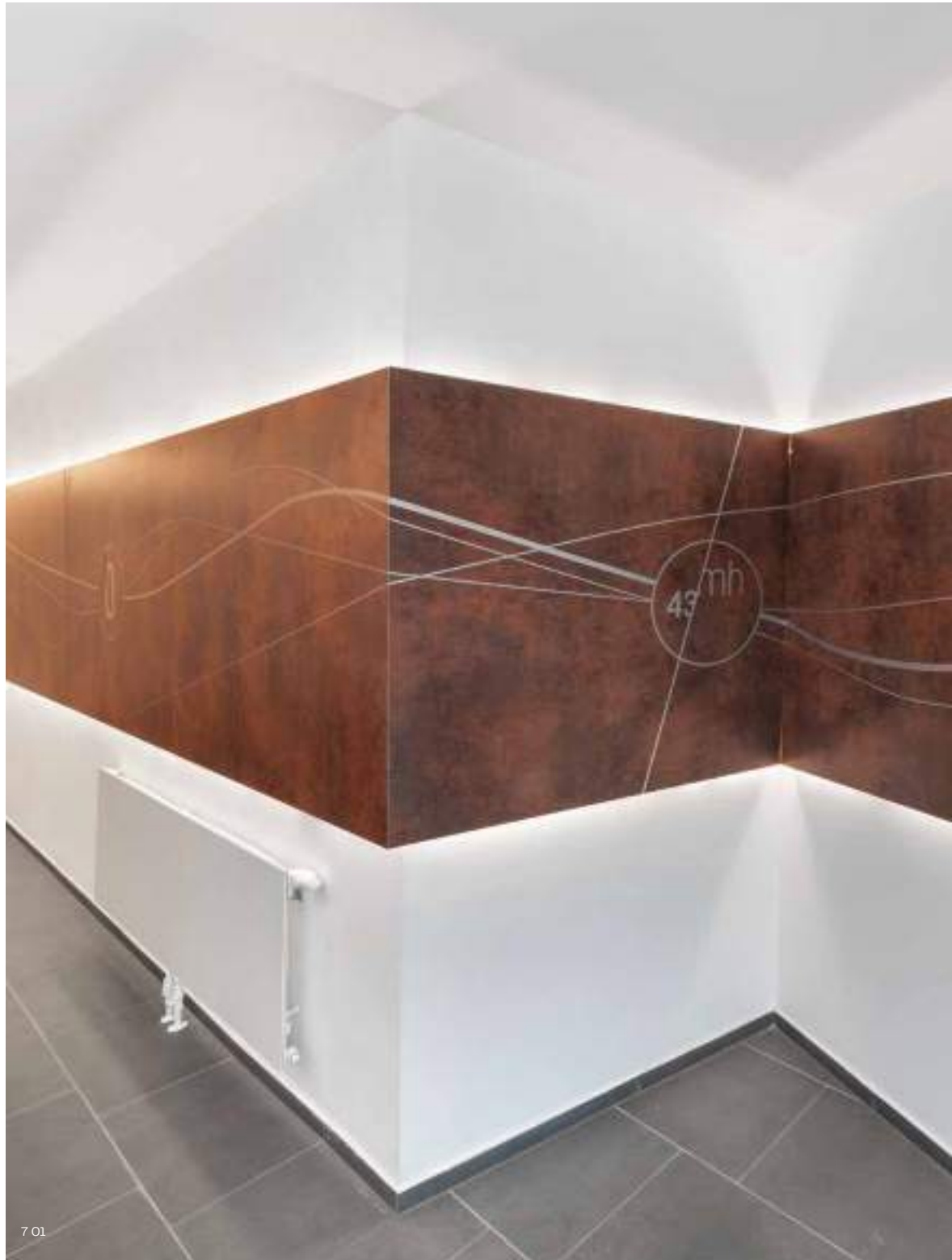
7 01 Decorative wall cladding with rear ventilation
